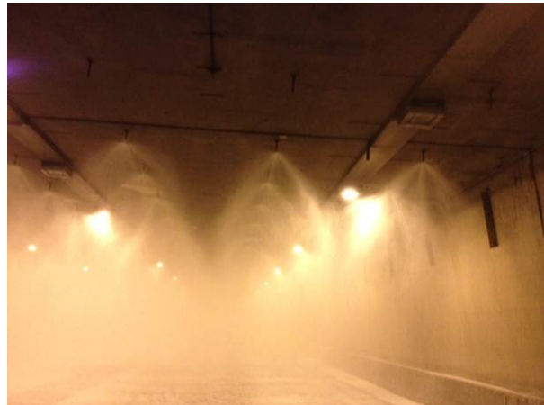
Fig.2: Activation of an FFFS deluge system in Mount Baker Tunnel (I-90) in Seattle (Source: IFAB)
