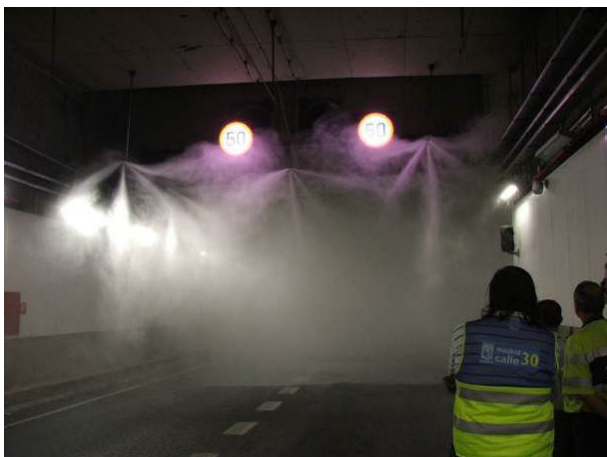
Fig. 1: Activation of a water mist FFFS in a tunnel on the M30 in Madrid (Source: IFAB)
